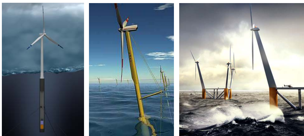
Figure 13. Concepts de turbines Hywind, Sway et Windsea.
