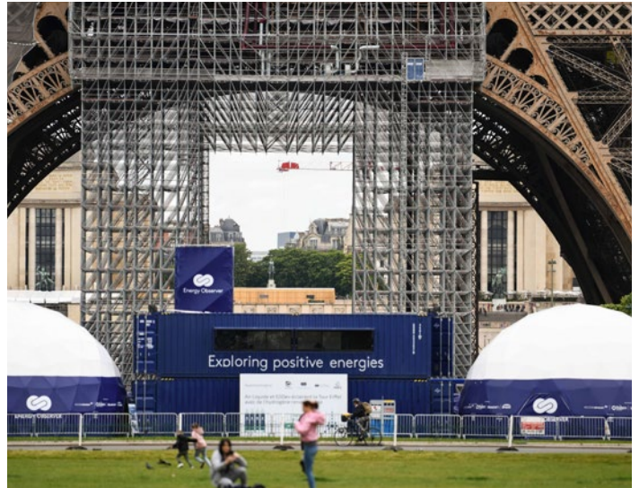
© Energy Observer Foundation – Thibaut Voisin
